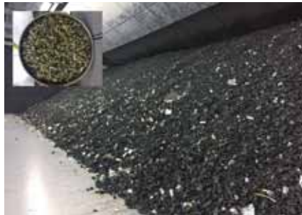
Over 18,000 lbs of lead was cleaned out of the recycled rubber berm in the indoor gun range.
